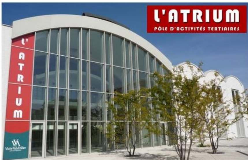
Figure 14 Façade de l'Atrium Source : http://www.vichy-economie.com/implanter-entreprise-vichy/zones-activites/atrium
